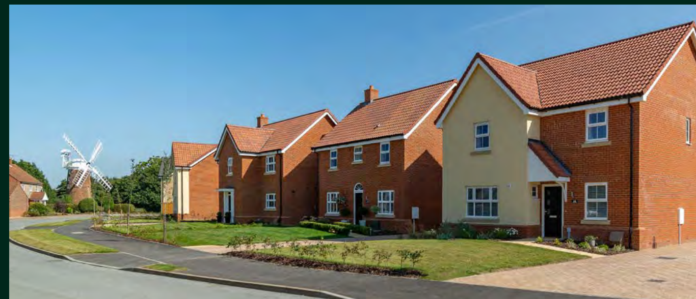
Mill View, Dereham
